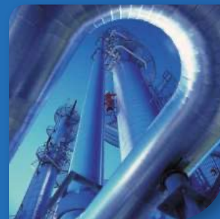
Chemical, Oil & Gas
